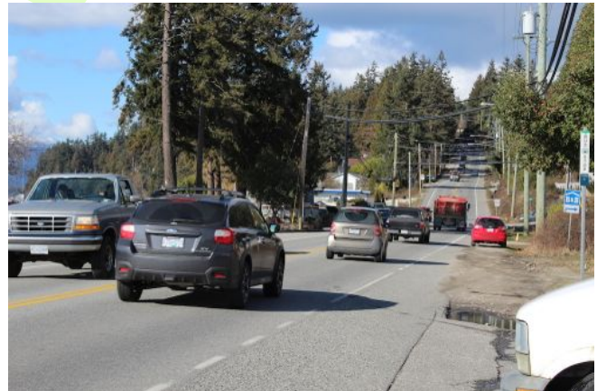
Narrow highway shoulder between Davis Bay and Sechelt.
